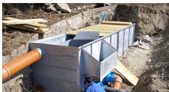
Illustration 7-4 Construction of a sedimentation basin in the mountains (HZI, n. y.)
