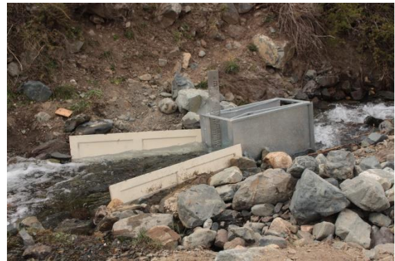
Illustration 6-2 Parshall flume
