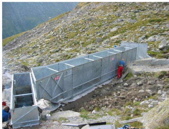
Illustration 7-3 Sedimentation basin for a Tyrolean weir in the mountains (HZI, n. y.)
