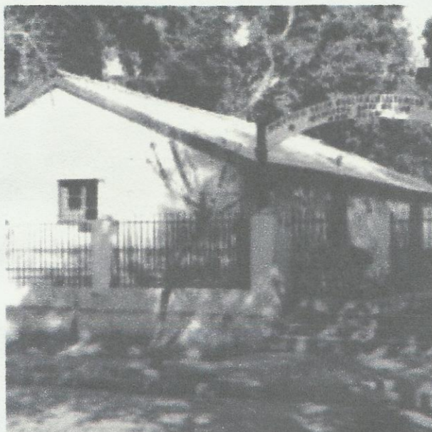
Hospital San Roque
